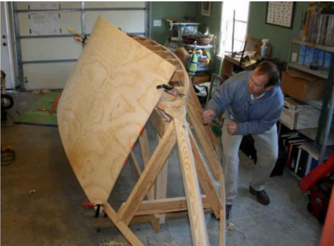
The plywood planking is temporarily clamped to the framing so that the frames can be used as a pattern to trace out the plywood shapes. This is a much more accurate way of cutting out the plywood than any pre-measuring method.
