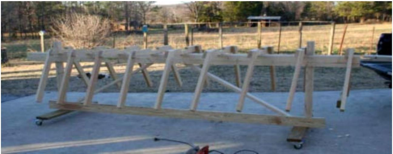
The frames are then assembled to the strongback jig and temporarily attached in-place.
