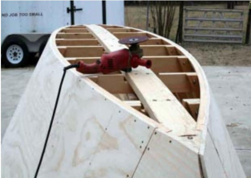
on the inside of the hull. This is simply a 6" wide block of the same thickness as the planking glued and screwed to the inside of the hull to form the joint. Here the side planking has been completed and is ground smooth to get ready to attach the bottom planking. All of the plywood planking is glued and screwed in-place.
