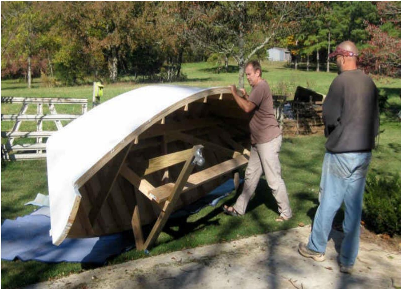
Time to flip over the hull and remove the strongback. After this, you just need to saturate the inside with epoxy resin to seal it and build out seats, center consoles, decking, sail rigging or whatever other accessories you wish.
