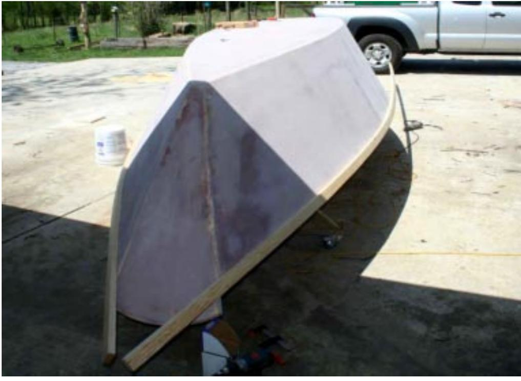
The rub rails are added next. These go on top of the fiberglass because they're there to deflect bumps and may need to be occasionally replaced.
